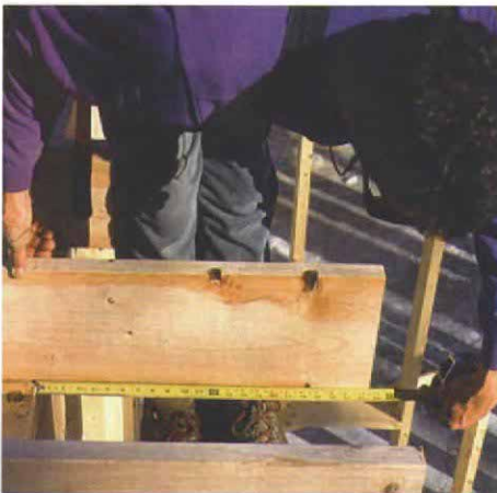
Setting the overhang. With a 2-ft. cantilever, the longest joists overhang 22½ in. The joists are then tacked in place.
